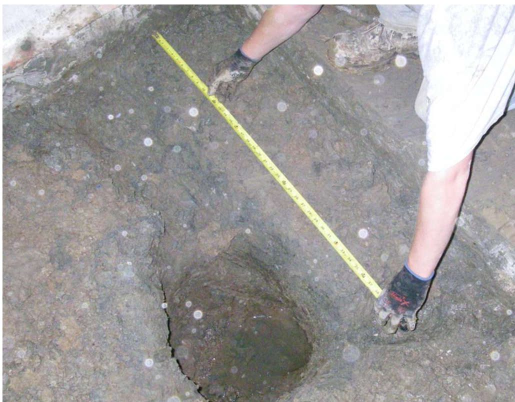
Figure 1: Measuring the exposed column footing for dimensions.
