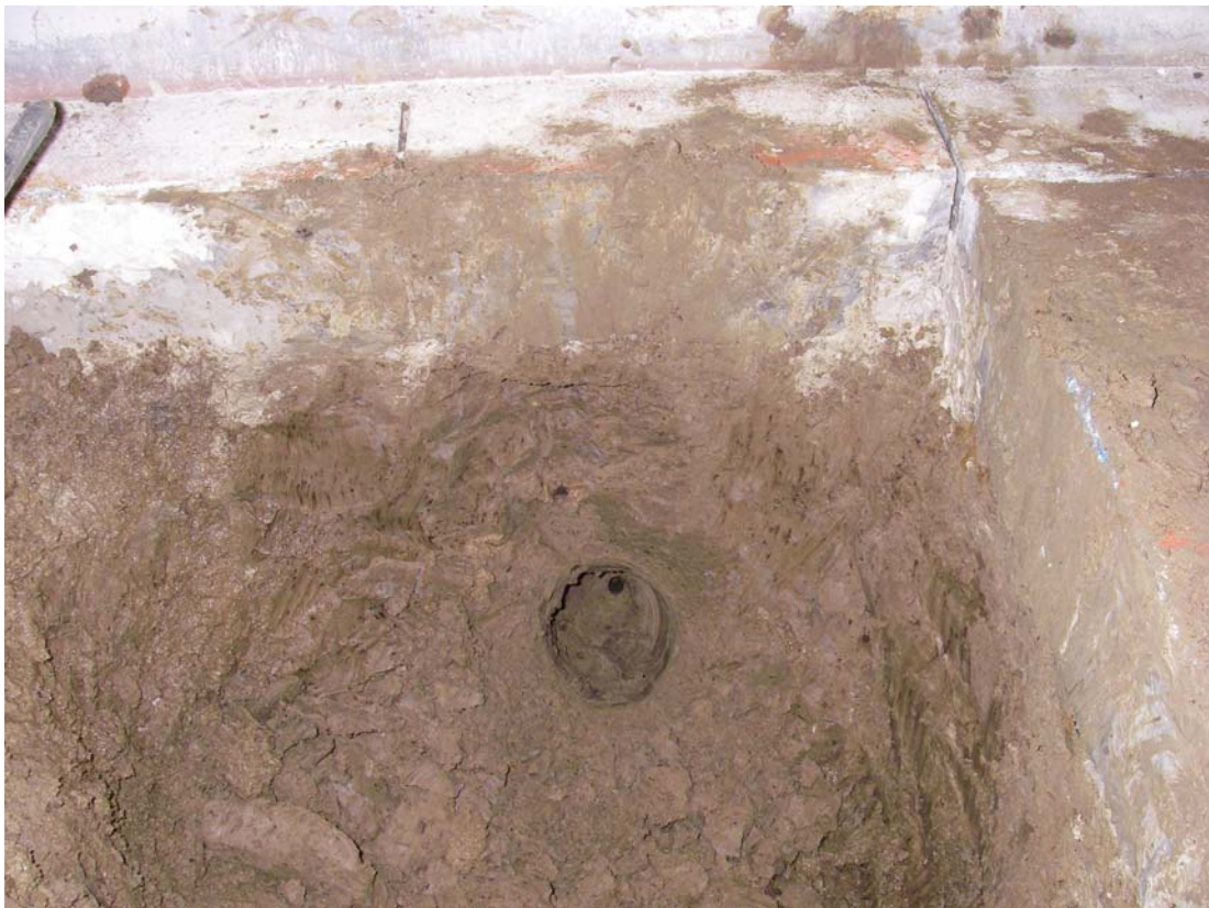
Figure 5: Excavation along the west edge (auger and tile probe holes seen above)
