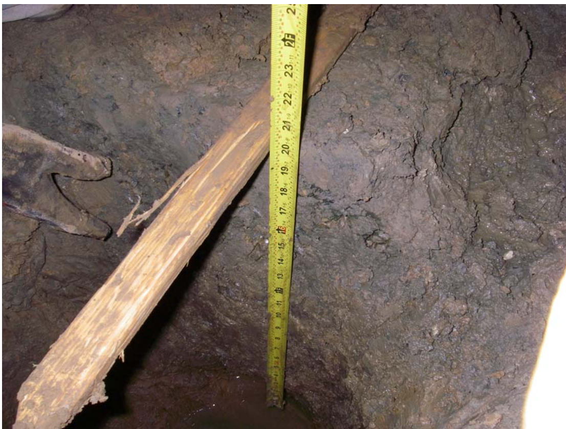
Figure 4: Depth to bottom of column footing
