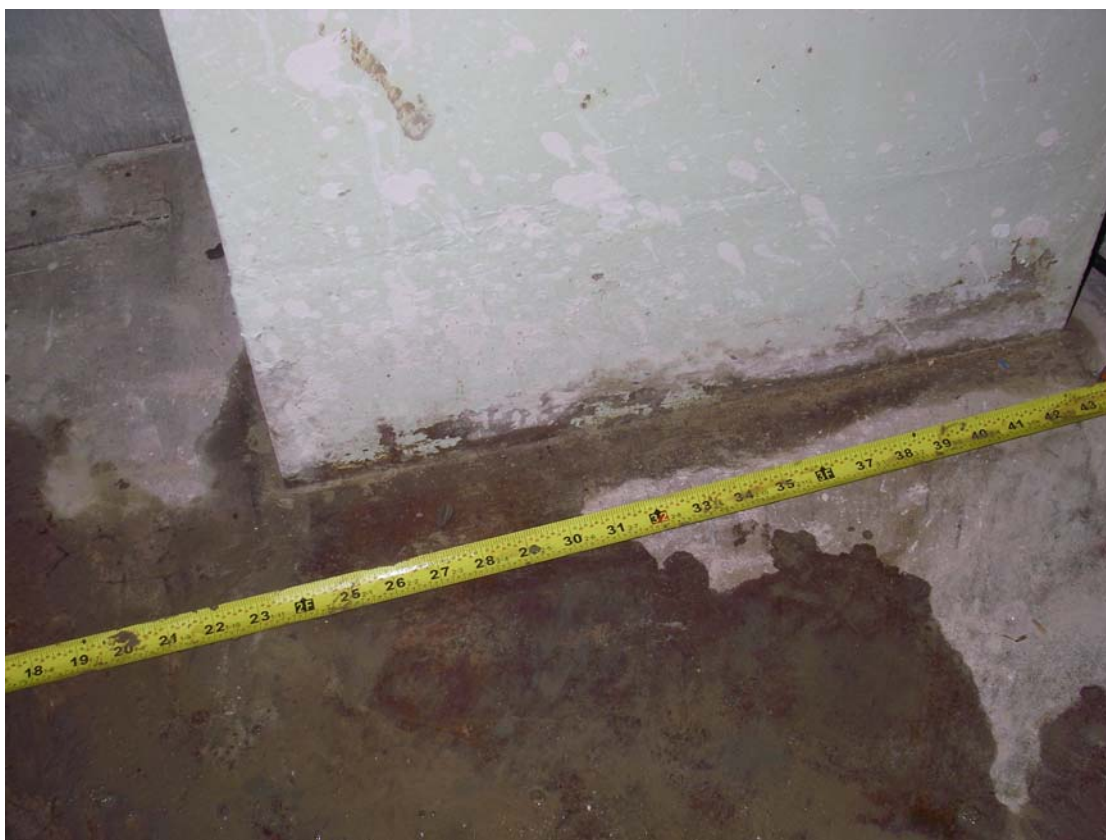
Figure 3: The distance from the edge of column footing to the center of column
